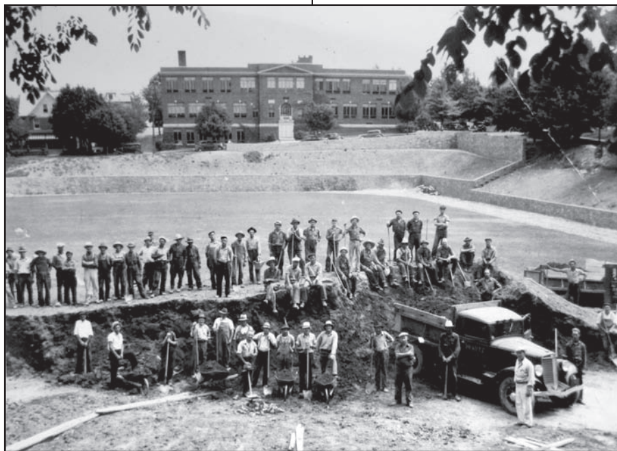
Works Progress Administration workers during the construction of Memorial Field, circa 1937. Photo provided.
